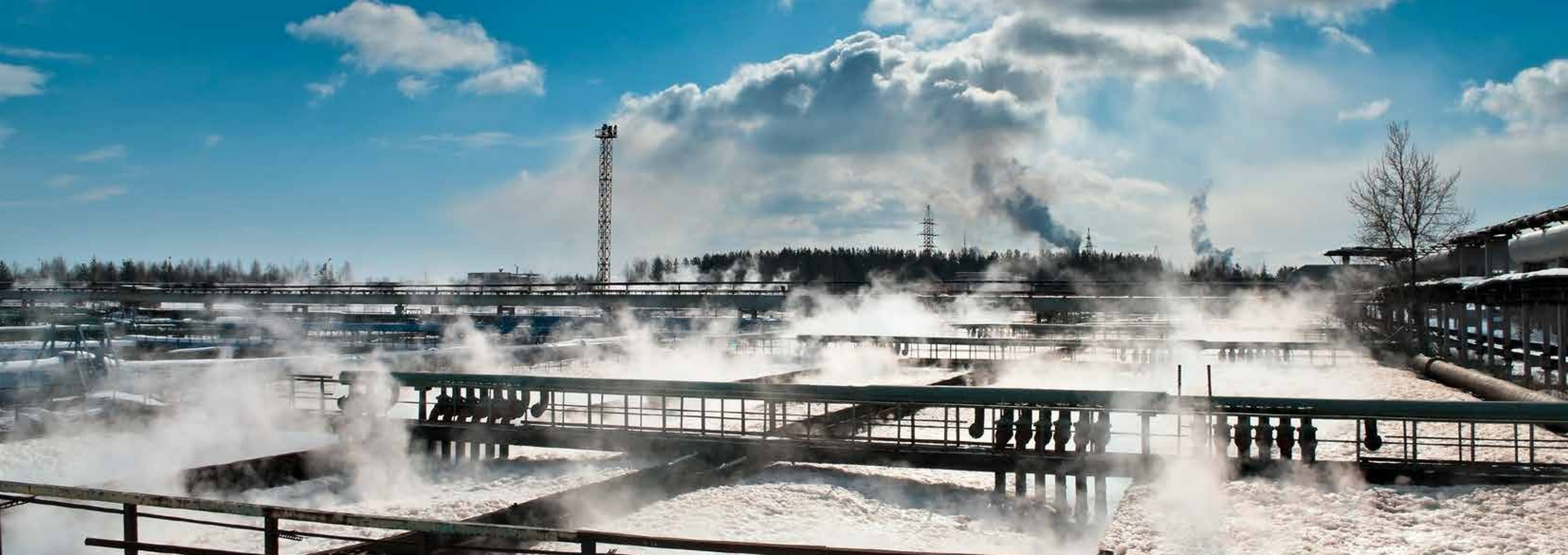
Wastewater treatment at a biological station.
